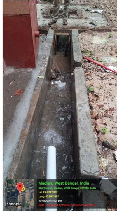
Fig 5: Rain water flowing into recharge chamber.
