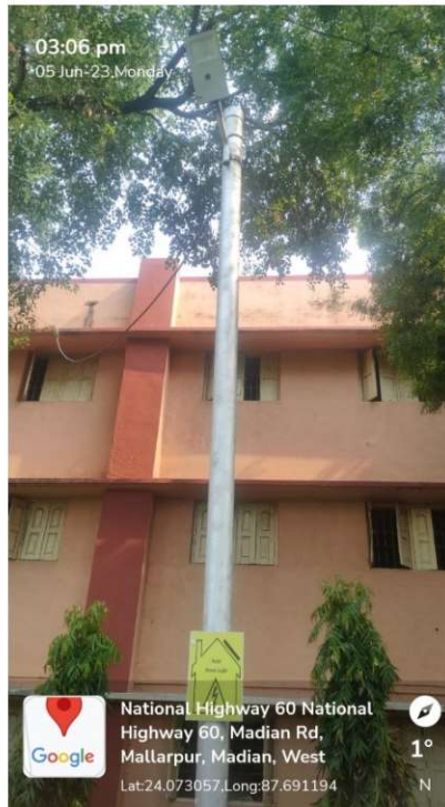
Figure 1d: The street light has been installed in the South-West side of the institution in front of the canteen building.
