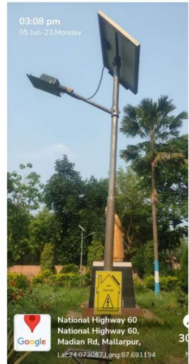
Figure 1d: The street light has been installed inside the Butterfly Garden situated in front of the institution.
